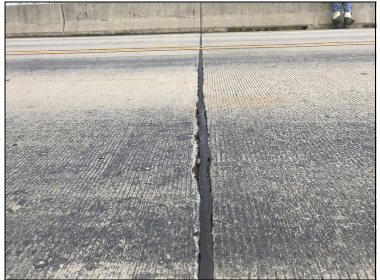
Bent #2 expansion joint-Adhesion failure.
