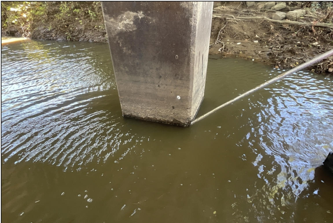
Bent # 2. Column # 1. Heavy abrasion at the water elevation.
