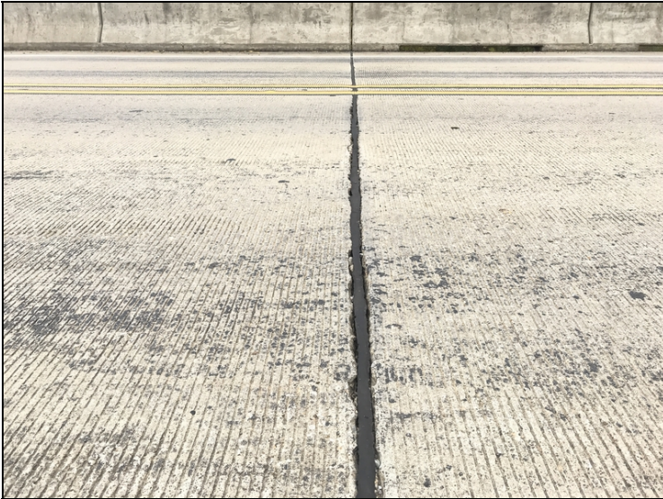
Bent #3 expansion joint adhesion failure.
