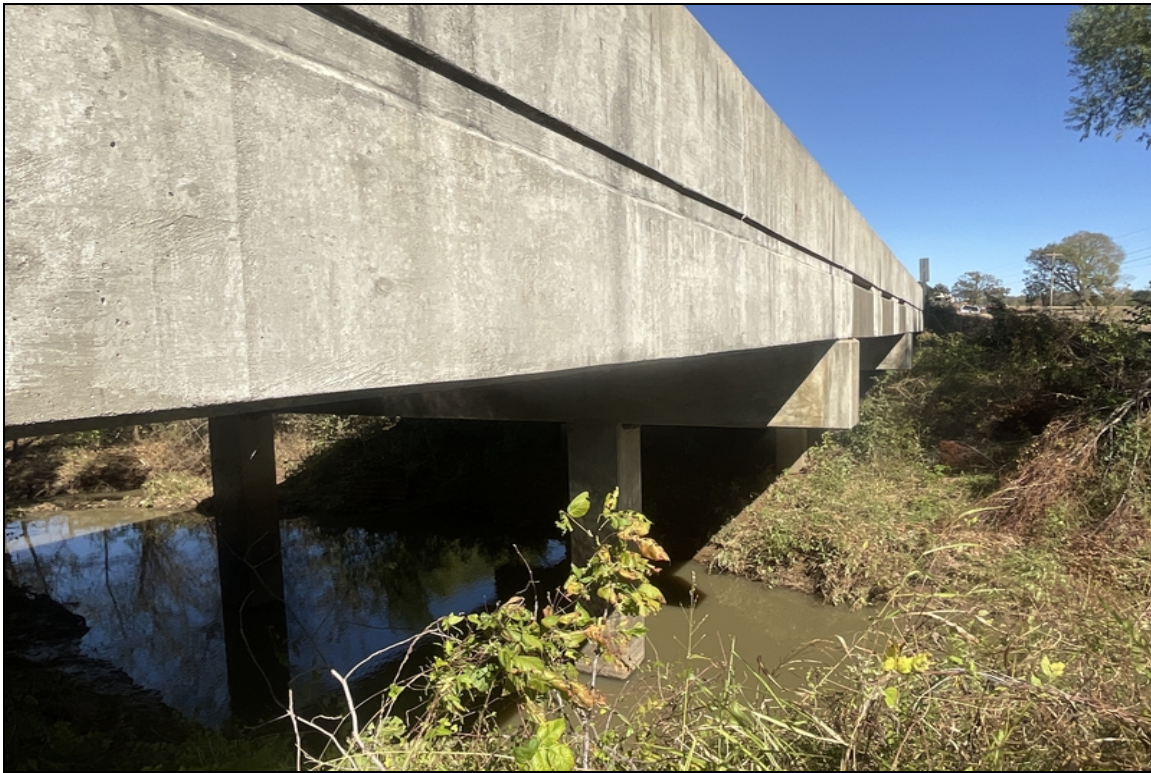
Slight creep visible in the edge of the slab.
