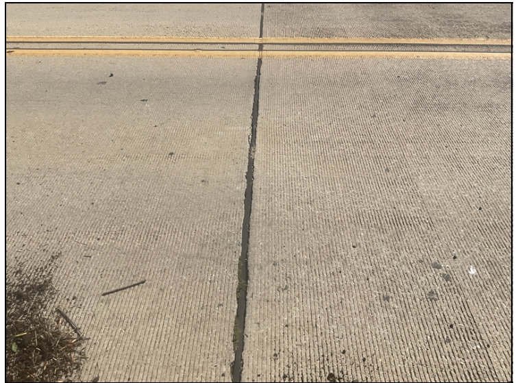
Expansion joint sealant over Bent # 3. Adhesion failure with leakage.
