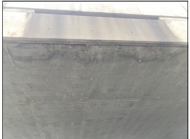
Span #2, right side-Delaminated areas along drip groove.
