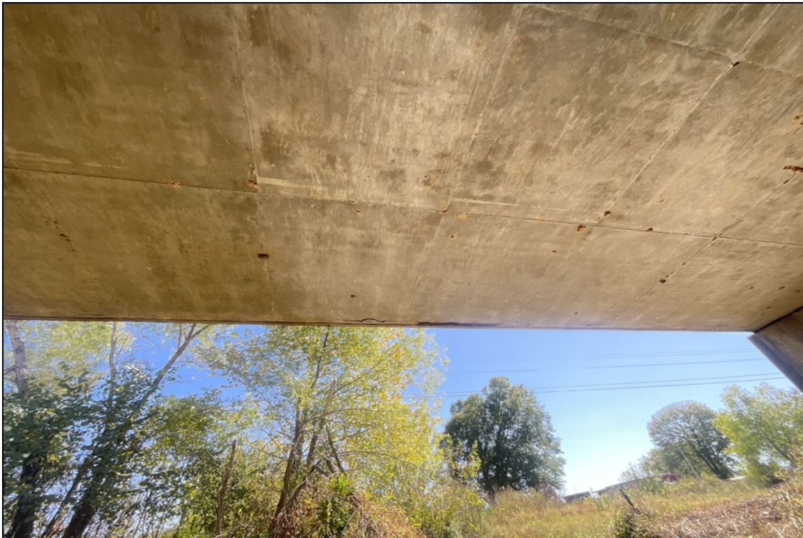
Undersurface of Span # 2 Right. Spalls with exposed reinforcing steel.
