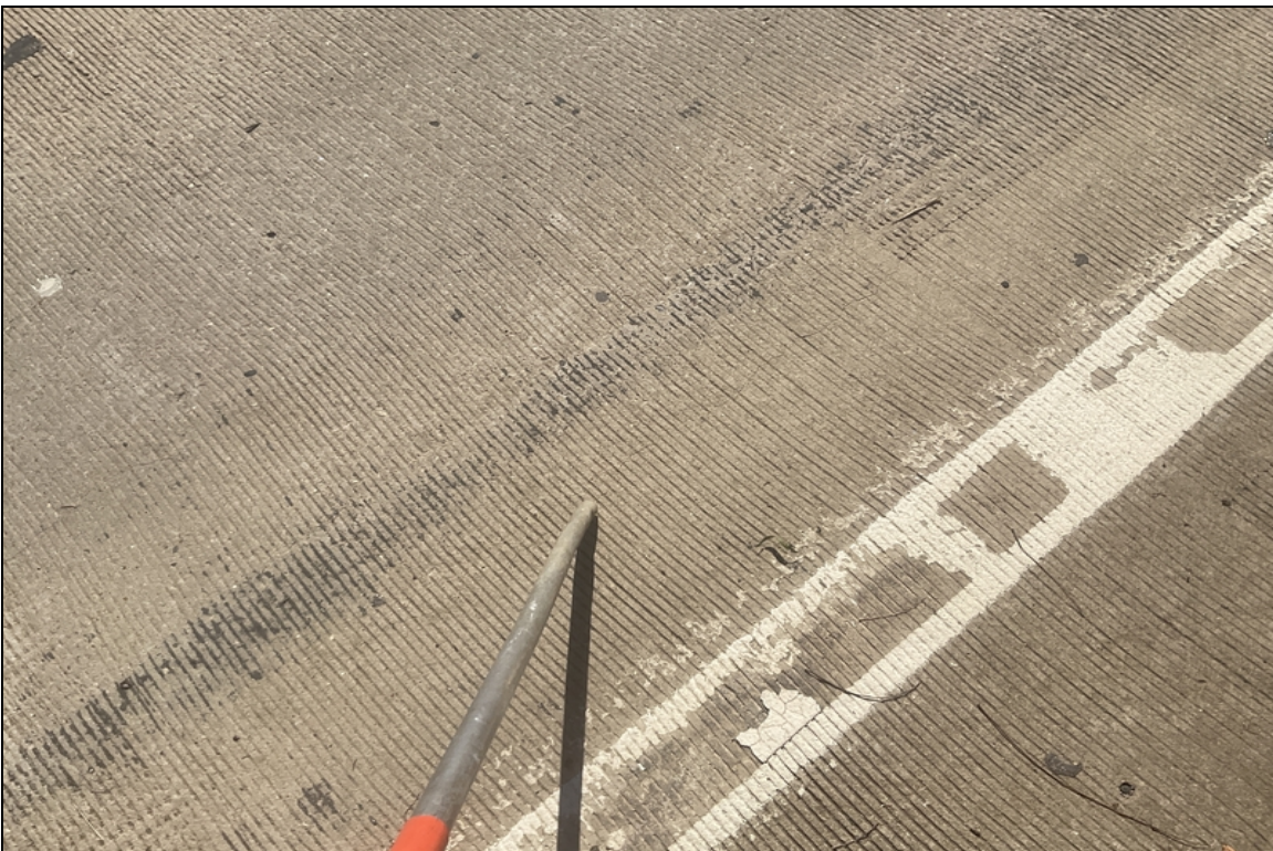
Longitudinal crack in Span # 1. Typical.
