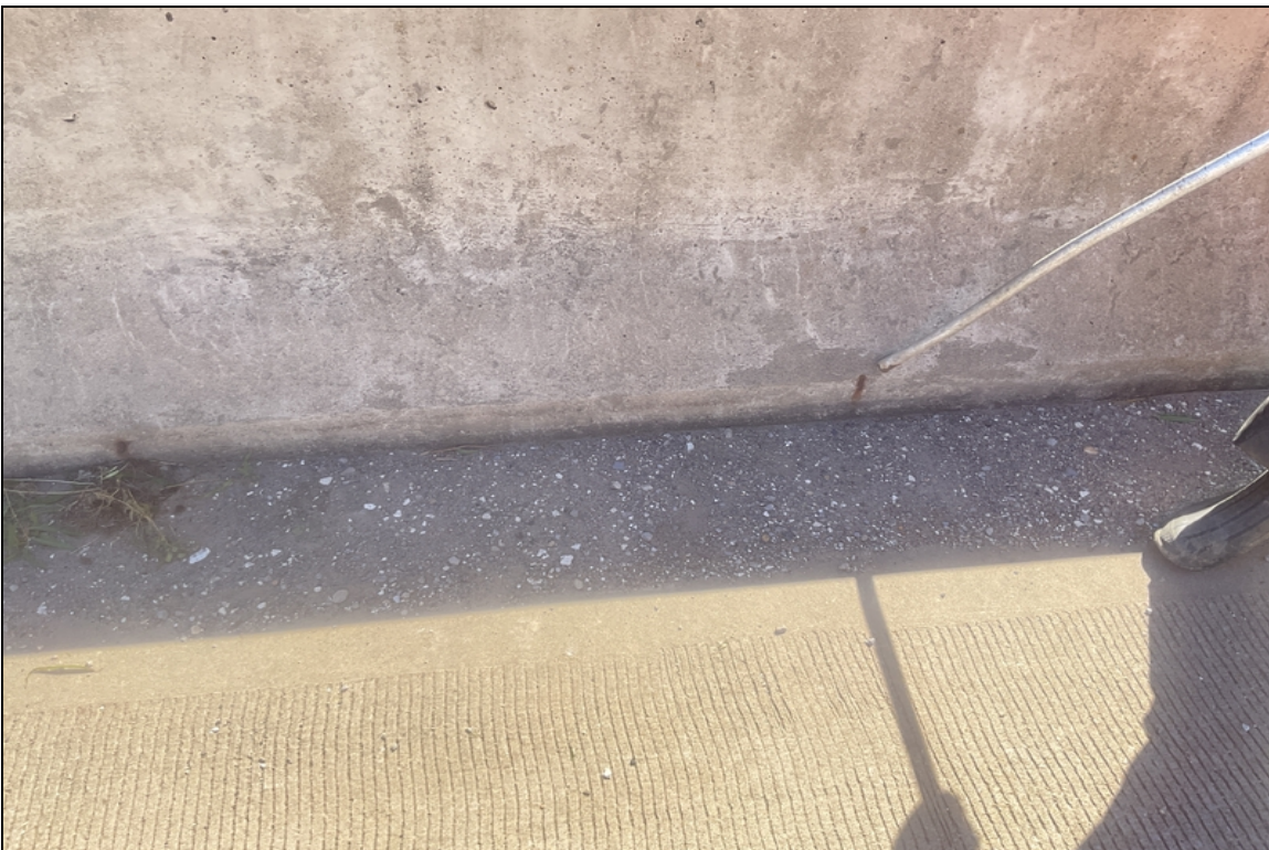
Spall with exposed reinforcing steel in the Right parapet of Span # 3.
