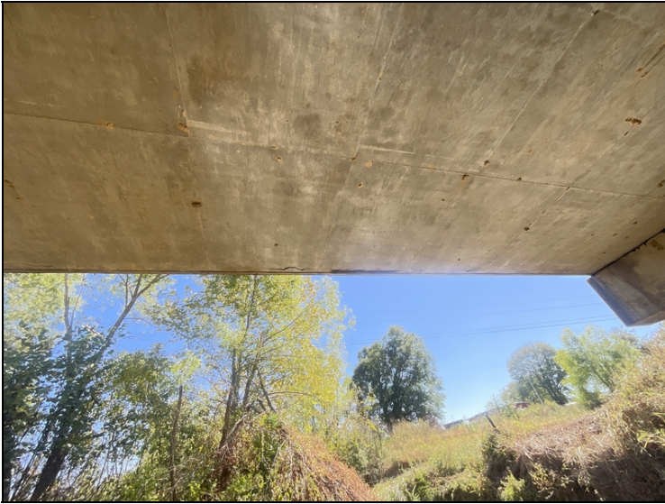
Undersurface of Span # 2 Right. Spalls with exposed reinforcing steel.
