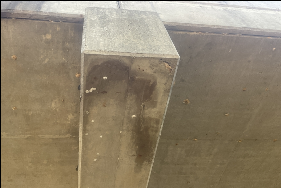
Bent # 2 cap. Left end. Undersurface has a shallow spall with exposed wood that appears to be chamfer cast in the concrete.
