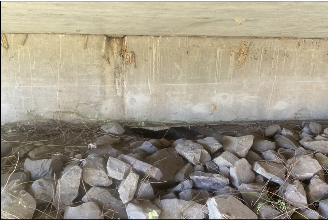
Bent # 1 with vermin holes under the abutment cap.
