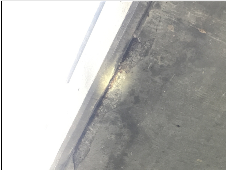
Span #2, right side-Spalling with exposed reinforcing steel along drip groove.
