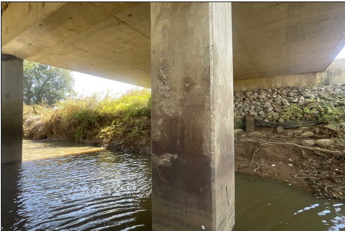
The ahead face of Bent # 2 Column # 1 has a 12" tall area of shallow spalling / concrete deterioration midway up the column.
