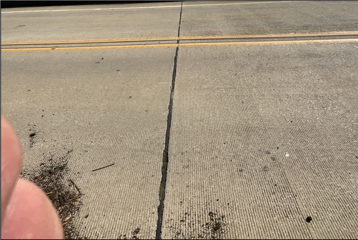
Expansion joint sealant over Bent # 3. Adhesion failure with leakage.
